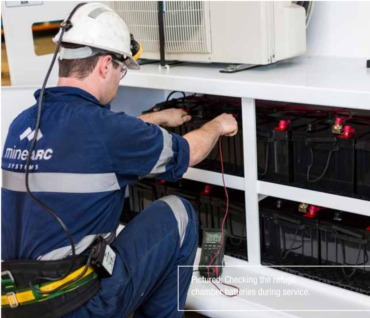
Pictured: Checking the refuge chamber batteries during service.
